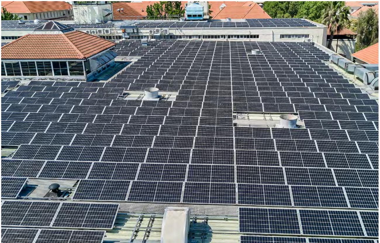
A 393 kW solar photovoltaic (PV) system on the roof of the Neelsie Student Centre. The power generated by the PV modules provides a third of the energy requirements of the student centre.
